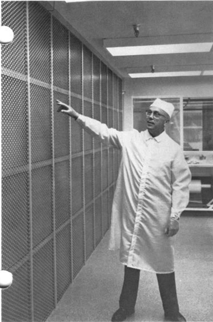
RAY ROBERTSON OF GARRETT-AIRESEARCH'S CLEAN ROOM STAFF INDICATES THE HUGE BANK OF ABSOLUTE FILTERS THAT COMPRISE ONE COMPLETE WALL OF THE LAMINAR FLOW CLEAN ROOM.
